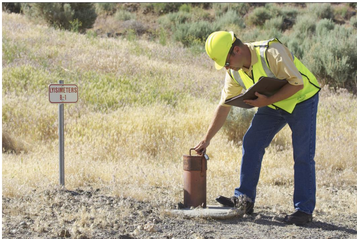
Figure 10 A technician checks a gas well at Lockwood landfill. (WM photo)
